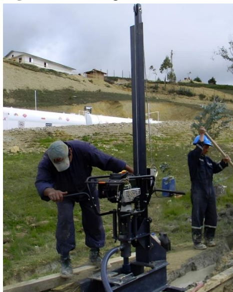
Figure 5. Piercing of the Piezometer
