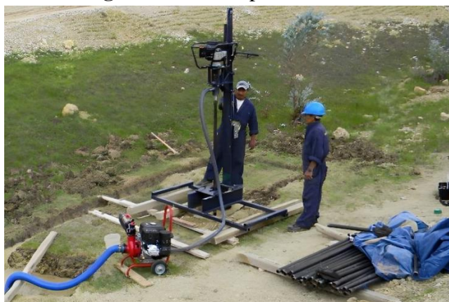
Figure 6. Blind Pipe Installation
