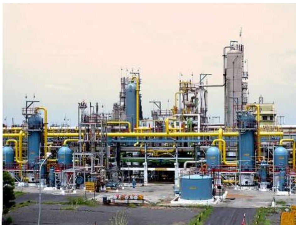
Fig.5. ONGC - Hazira (Gujrat) green hydrogen plant 9
