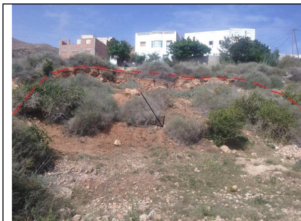
Photo 1 : Rotational landslide affects Eo-oligocene marls in the Boujibar district.
