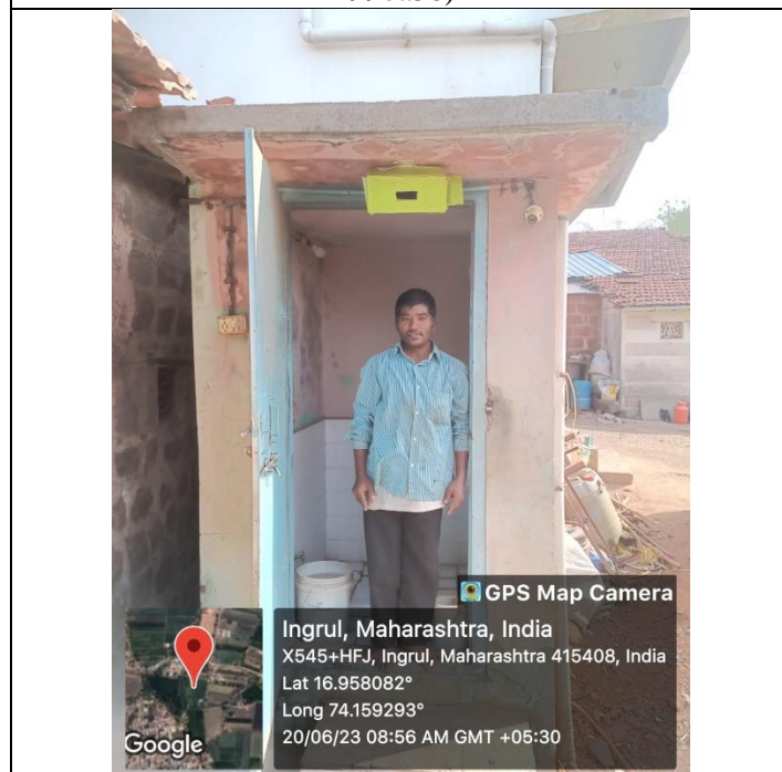
Sensor Attached in the toilet
