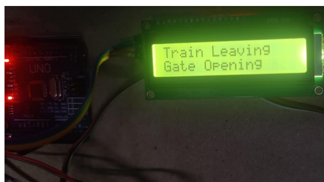
Fig.15: Showing Gate opening while Train leaving the Gate
