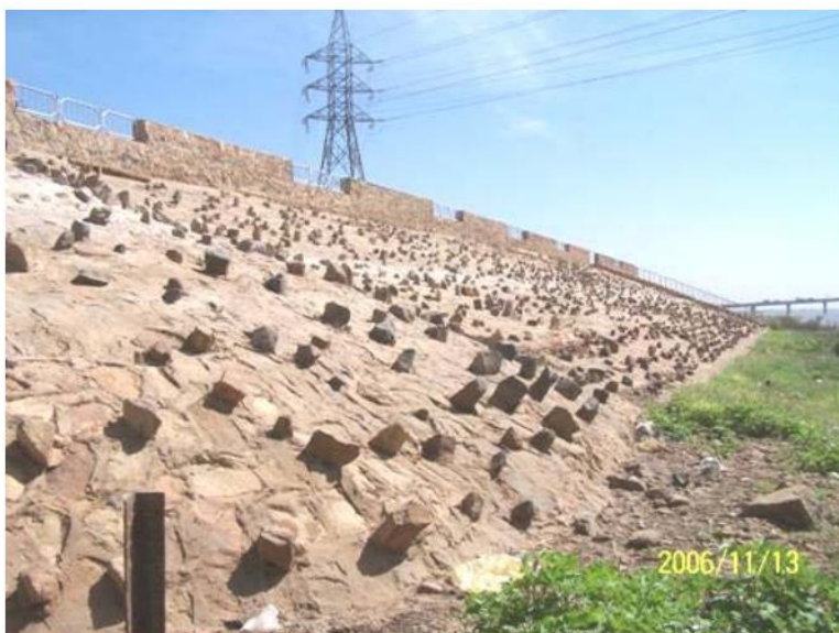
Fig. 2 Hardened bank is roughened by sticking stones on the surface on the Blue Nile River in Sudan
