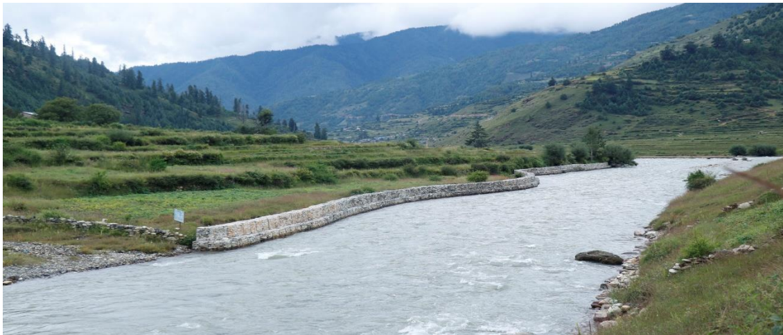
River bank training constructed by NCCSP
