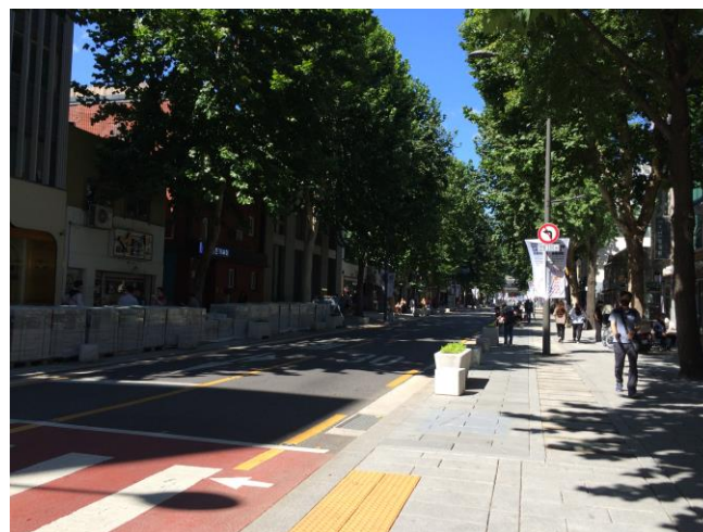
Fig.18 The wide pavement for pedestrians
