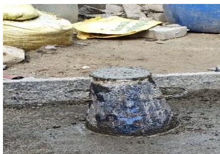
Figure 3: Slump test (Before)
