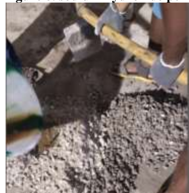
Figure 10. Geopolymer concrete mixing
