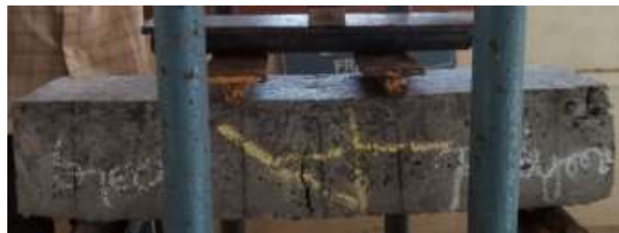
Figure 16. Failure of prism
