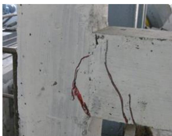
Figure.10 (PP 75% +Steel 25% ) 2.0 BC Joint Failure Mode
