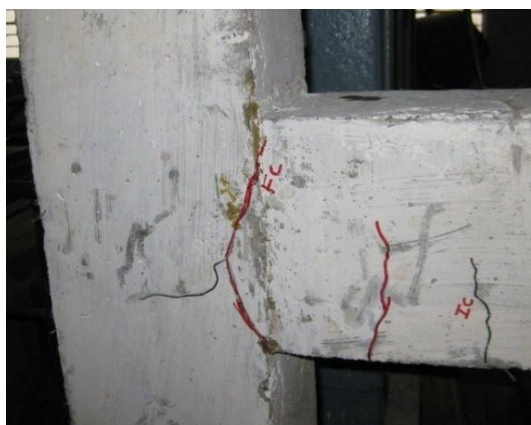
Figure.8 Failure Mode - Typical Concrete BC Joint
