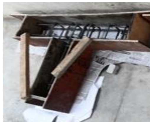
Figure.4 Reinforcing of the BC Junction
