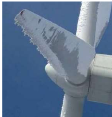
Figure 11. Ice accumulation on wind turbine blades.
