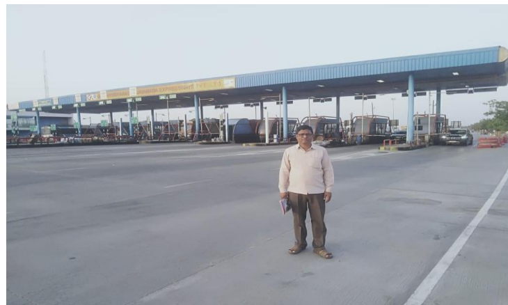
Fig 4 View of Korlapahad Toll Plaza on NH65
