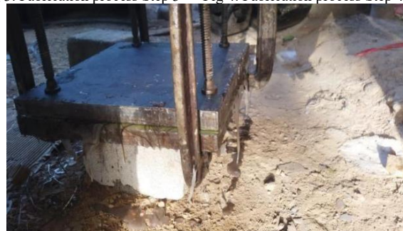
Fig 5: fabrication process step 5
