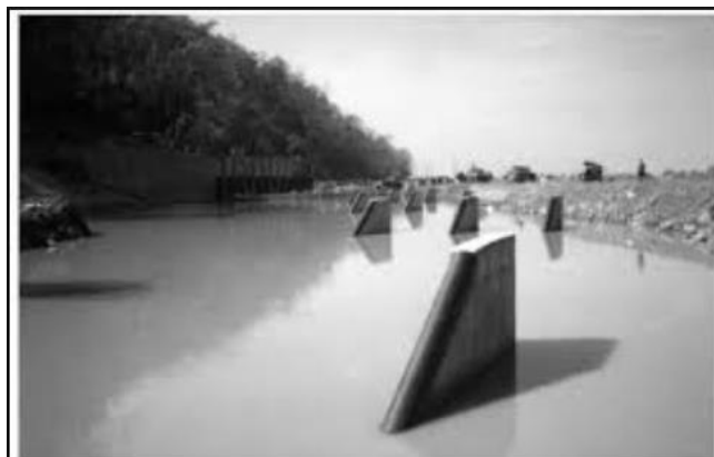
Fig.13 Aligned Submerged Vanes
