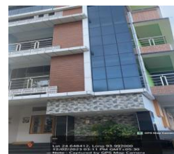
i) Typical picture of RCC House
