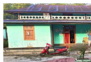
iii) Typical picture of AT mud house
