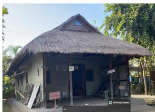
v) Typical picture of AL earthen house (Meitei Yumjao)
