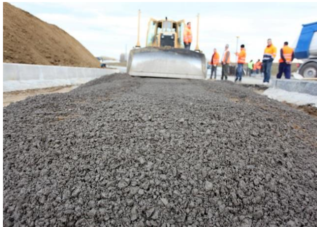
Fig-7: Asphalt Modified with Rubber Powder
