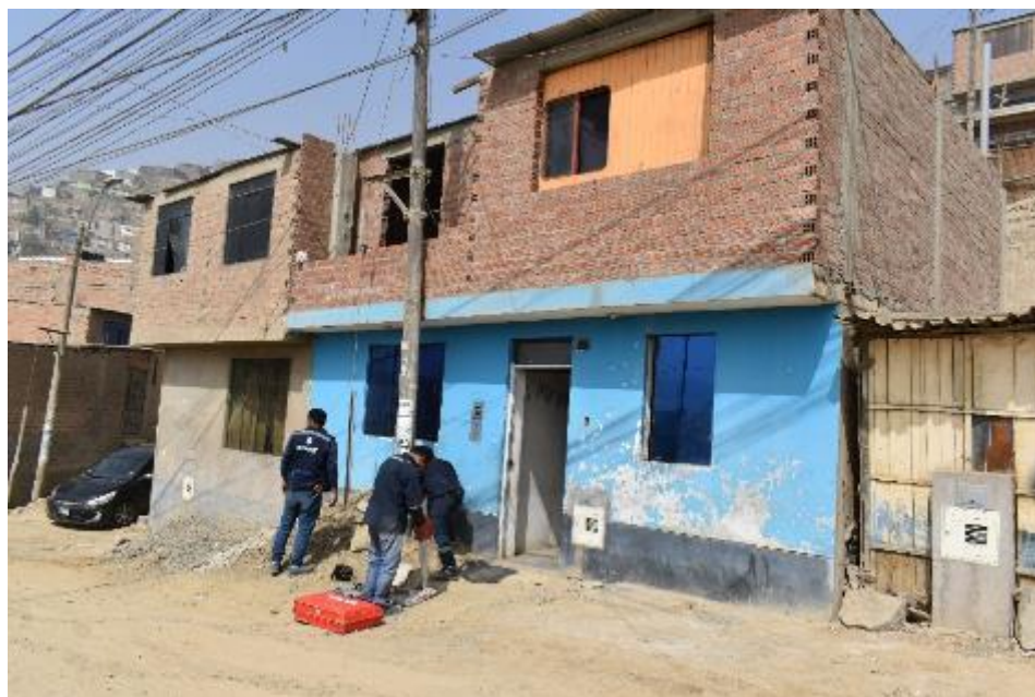
Figure 5. Image of the operating personnel specialized in cylindrical coring.
