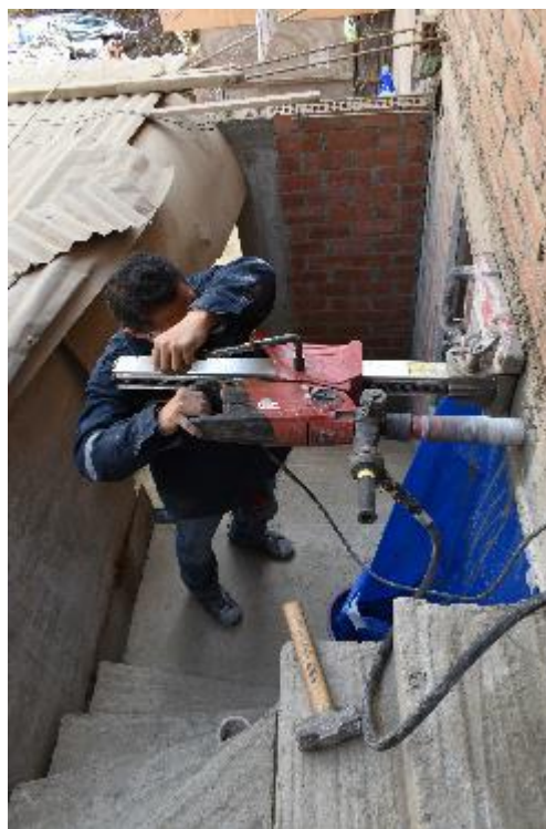
Figure 7. Core extraction process.
