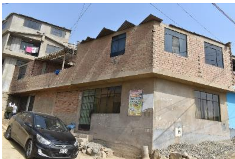
Figure 11. Façade view. Quispe Blaz family.
