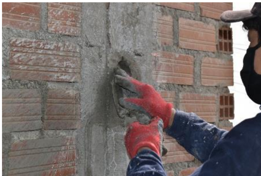
Figure 9. Repair process of the extracted cylindrical core.
