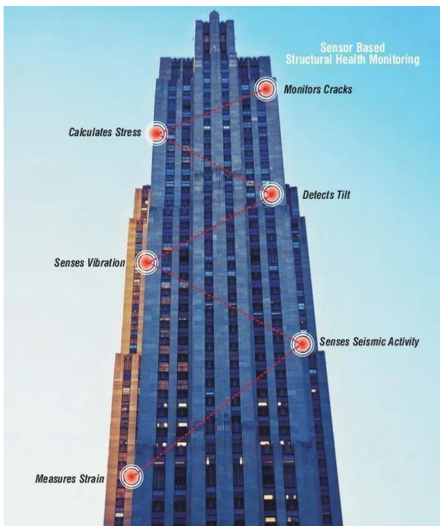
Figure 1.1 Sensor based Structural Health Monitoring
