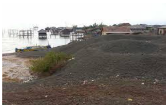
Figure 2. Nickel slag as a backfill on the beach
