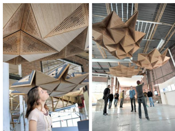
Figure 7: Ceiling resulted from the singling of the variable acoustic geometry study ball at the University of Michigan. (Furuto, 2012)
