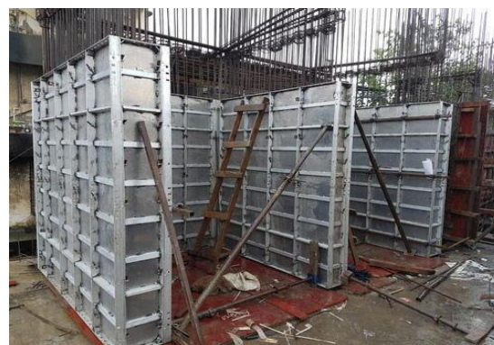
Fig 3: Aluminum/ Mivan Formwork
